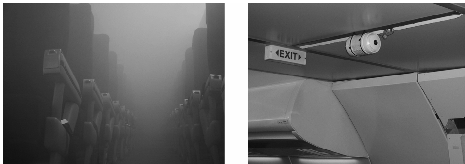
Figure 13: Test Installation of Acoustic Signalling Device
